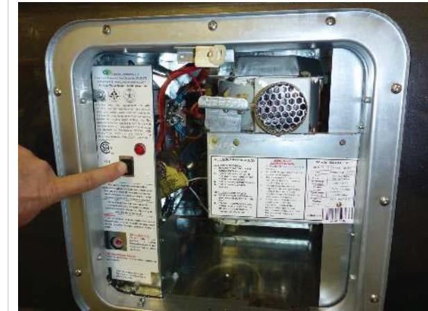
Turn off the water heater
